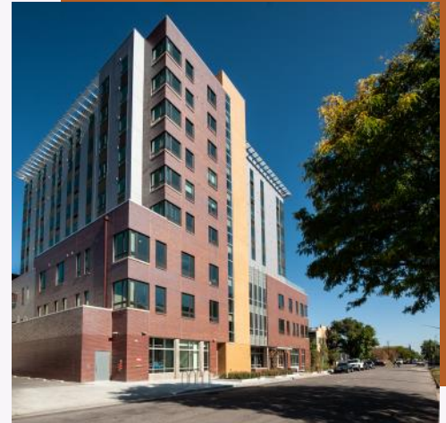
External photo of the new Renaissance Legacy Lofts and Stout Street Recuperative Care Center, located at 2175 California Street in Denver, Colo.
