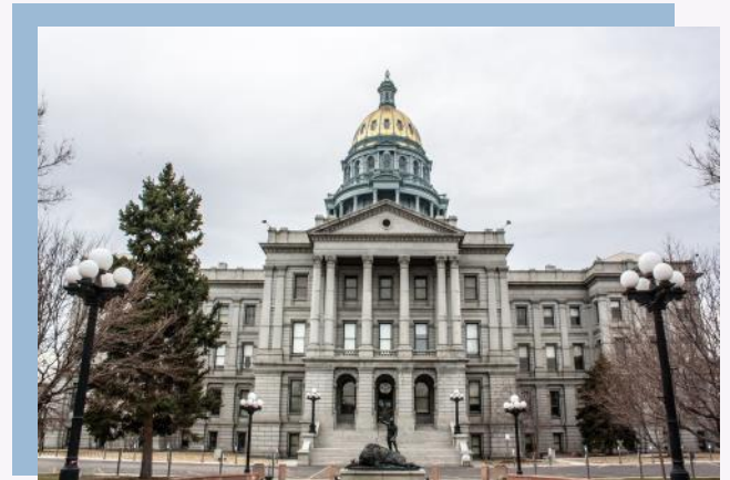
The Colorado Capitol building.
