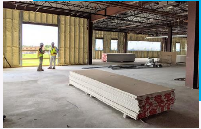
Construction at Pueblo Community Health Center's East-Side Expansion project
