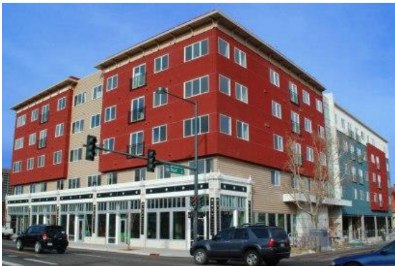
Renaissance Uptown Lofts, at the corner of Pearl and Colfax in Denver, is CCH's newest affordable housing development for formerly homeless and low-income residents.
